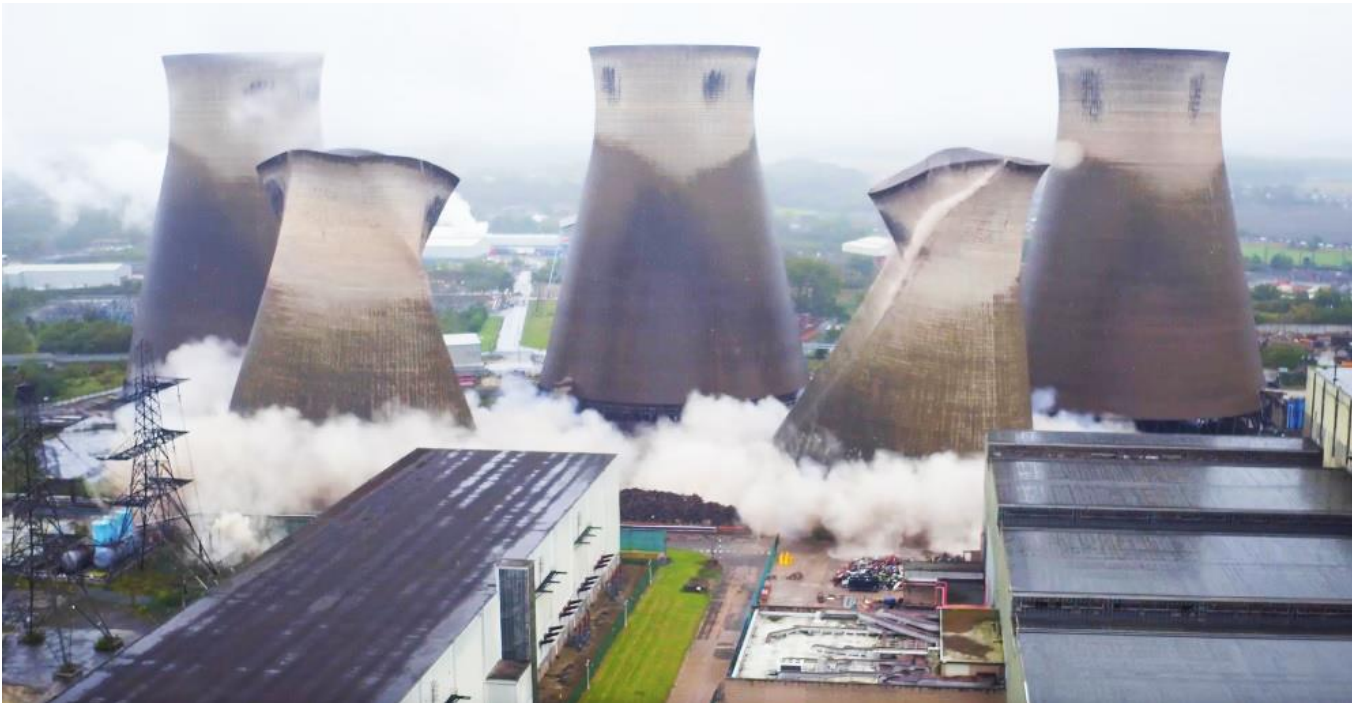
Ferrybridge - Power Station Cooling Towers
